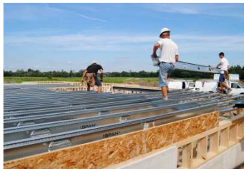
Figure 1 - TotalJoists are comparable in weight to I-Wood
