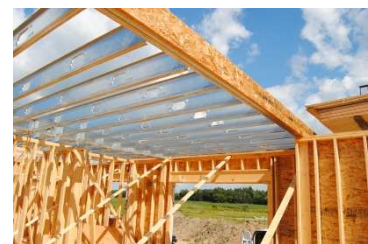
Figure 2 - TotalJoist integrate well into wood framed structures
