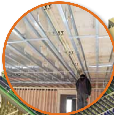
Running Services in Floor Assembly
