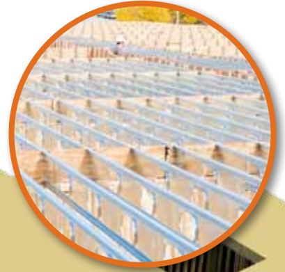
Installing Roof Joists
