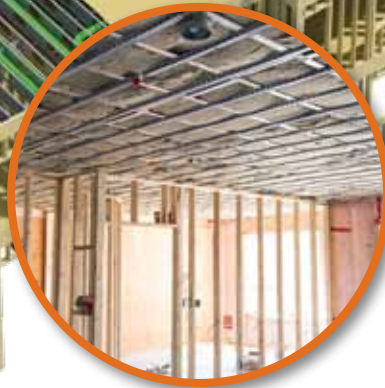
Ceilings Ready for Drywall
