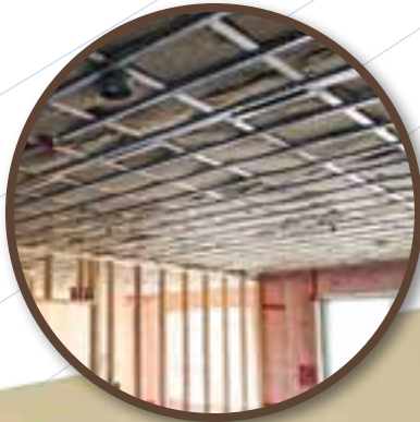
Ceilings Ready for Drywall
