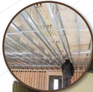
Running Services in Floor Assembly
